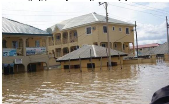
Fig. 4b) Abuja flooding swiped away five family, (FCT) North-Central Nigeria
