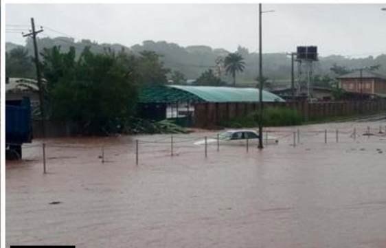
Fig. 4e) Kano city flooding due to blocked drainage system after heavy rainfall, North-Western Nigeria
