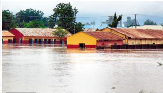
Fig. 4d) Bauchi flooding due to blocked drainage system after first rainfall, North-Eastern Nigeria
