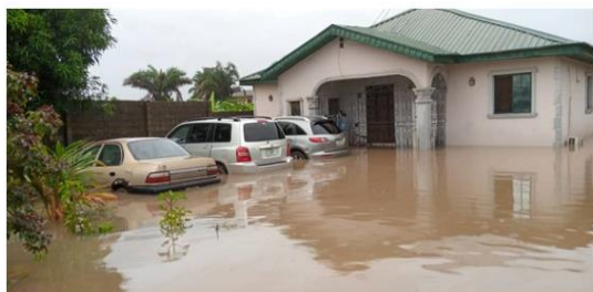
Fig. 4a) Flash flood incident at Ikorodu-Sagamu road Lagos state, South-Western Nigeria
